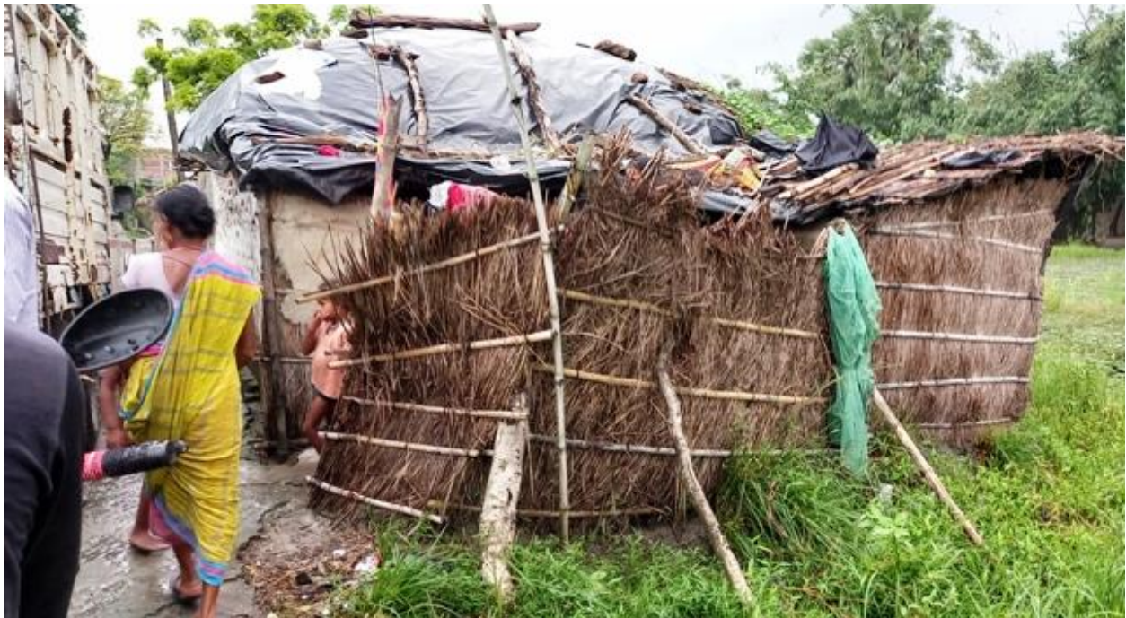
Pic 2.1: By flood damage house
